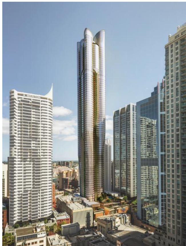
Figure 2 – FJMT tower viewed from the south-east
