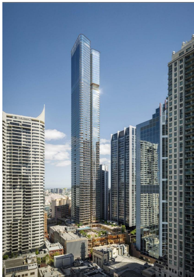
Figure 5 – SOM + Crone tower viewed from the south-east
